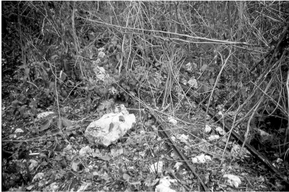
FIGURE 19.5. A section of rail line within the El Edén wetland.
